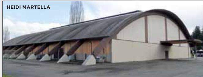
HEIDI MARTELLA Rainier Auditorium on the campus of Auburn Adventist Academy in Auburn, Wash., is warmer and more energy efficient after replacing single-pane windows with wood siding.
