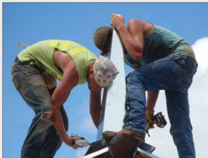
Adding a finishing touch, Colton Hayden and Logan Saterdal fasten the steeple to the newly completed Chilunguni Church in Malawi.
