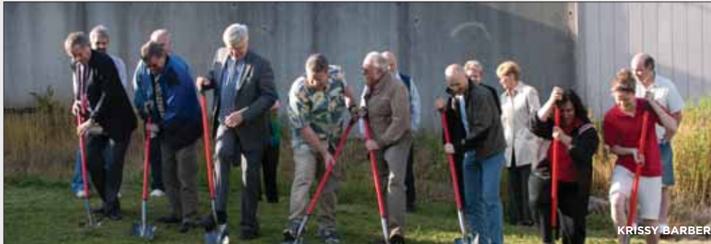
The Rivergate Adventist Elementary School and the Gladstone Park (Ore.) Church broke ground in 2009 on an expansion project to benefit both the school and the church.
