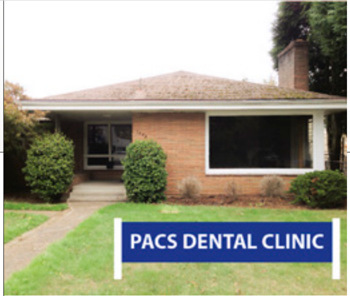
A sign superimposed in front of the house shows what it could look like once it has opened as the PACS Dental Clinic.
