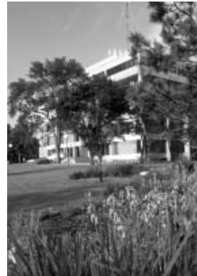
Everett Dick Building (UC’s Administration Building).
