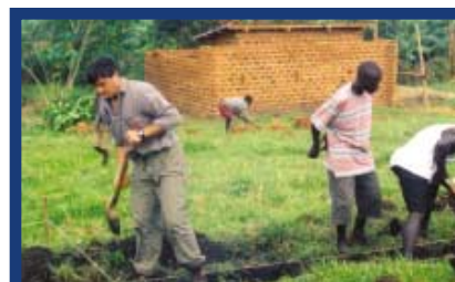
Volunteers help dig the foundation for the new orphanage.
