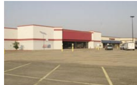
The Wal-Mart in New Iberia, La., donated their old store for a warehouse. This 150,000-sq.-foot facility is very much appreciated by everyone involved.
