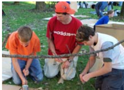
The freshmen constructed walls for temporary shelters.
