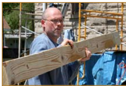
Gary Holman brings a board for a roof jack.
