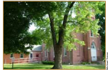
The Martinsville Church, the oldest church structure in Martinsville, is now a beautiful house of worship.
