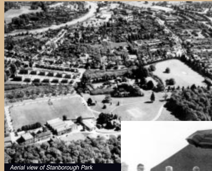
Aerial view of Stanborough Park
