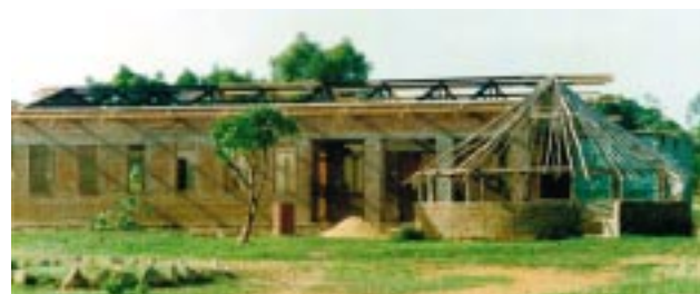
Juba Clinic, South Sudan, in the process of completion
