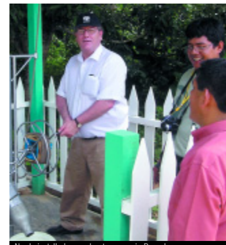
Newly installed ground water pump in Pucallpa
