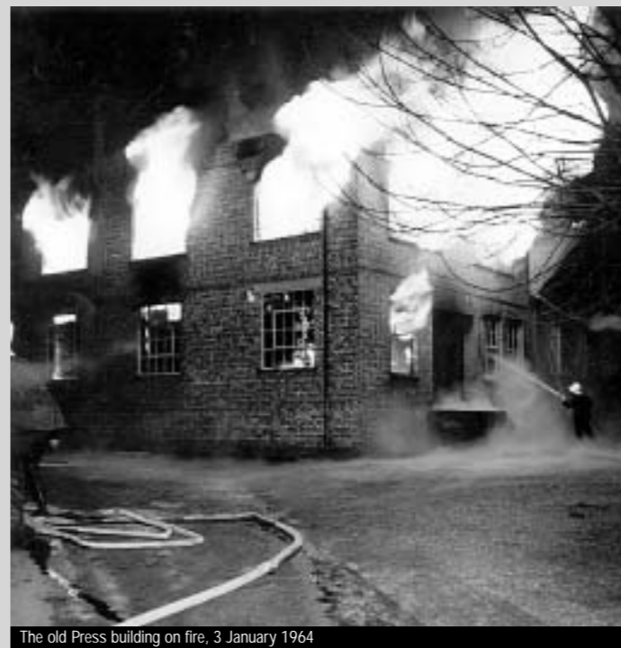
The old Press building on fire, 3 January 1964
