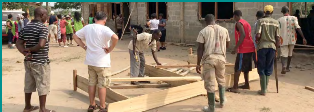
ADRA-UK volunteers and ADRA Ghana refurbishing the classrooms
