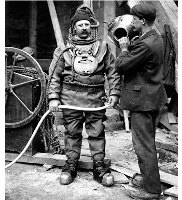
William Walker is seen here being dressed by an aide. His total gear weighed in excess of 90 kgs. Once prepared, he had to climb down 13ft to the Cathedral foundations. Photo by John Crook.
