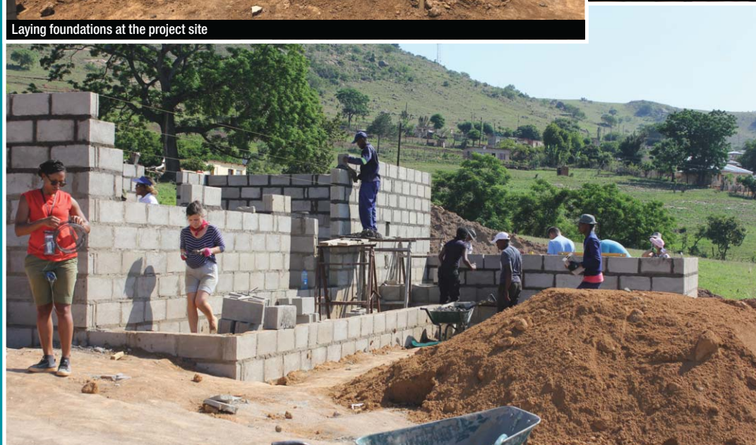
Pre-school halfway through its build
