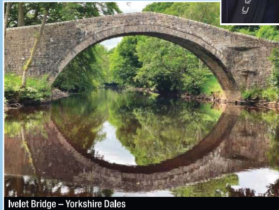
Velet Bridge – Yorkshire Dales
