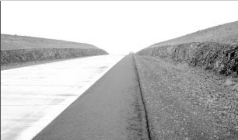
FIGURE 5. A long road cut showing the smooth contact between the basalt and the overlying loess. There was 10-20 cm of gravel between the top of the basalt bed and the loess.
