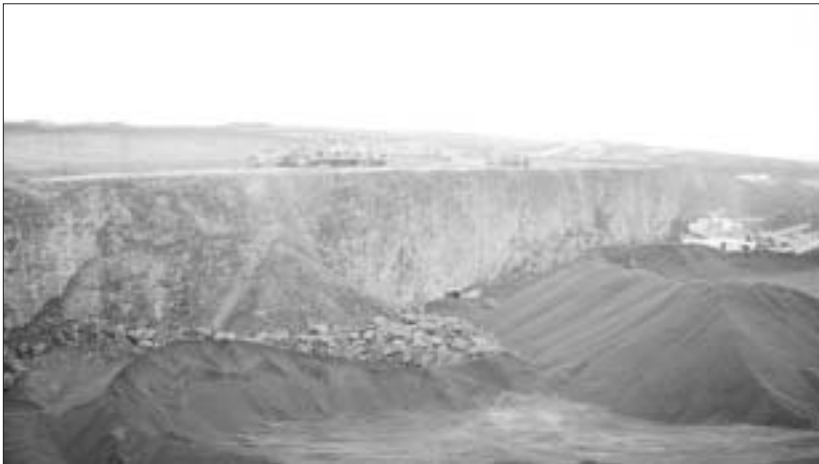
FIGURE 2. At Site 26, the equipment is sitting on the smooth, flat surface of the basalt. The loess, visible in the background, has been removed.
