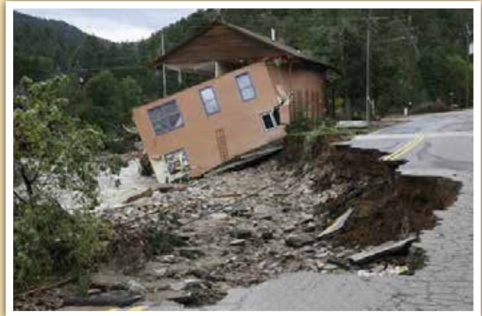
A wall clings to the remnants of a house in Jamestown, Colorado after a flash flood destroyed much of the town. PHOTO: RICK WILKING/REUTERS, WASHINGTONPOST.COM
