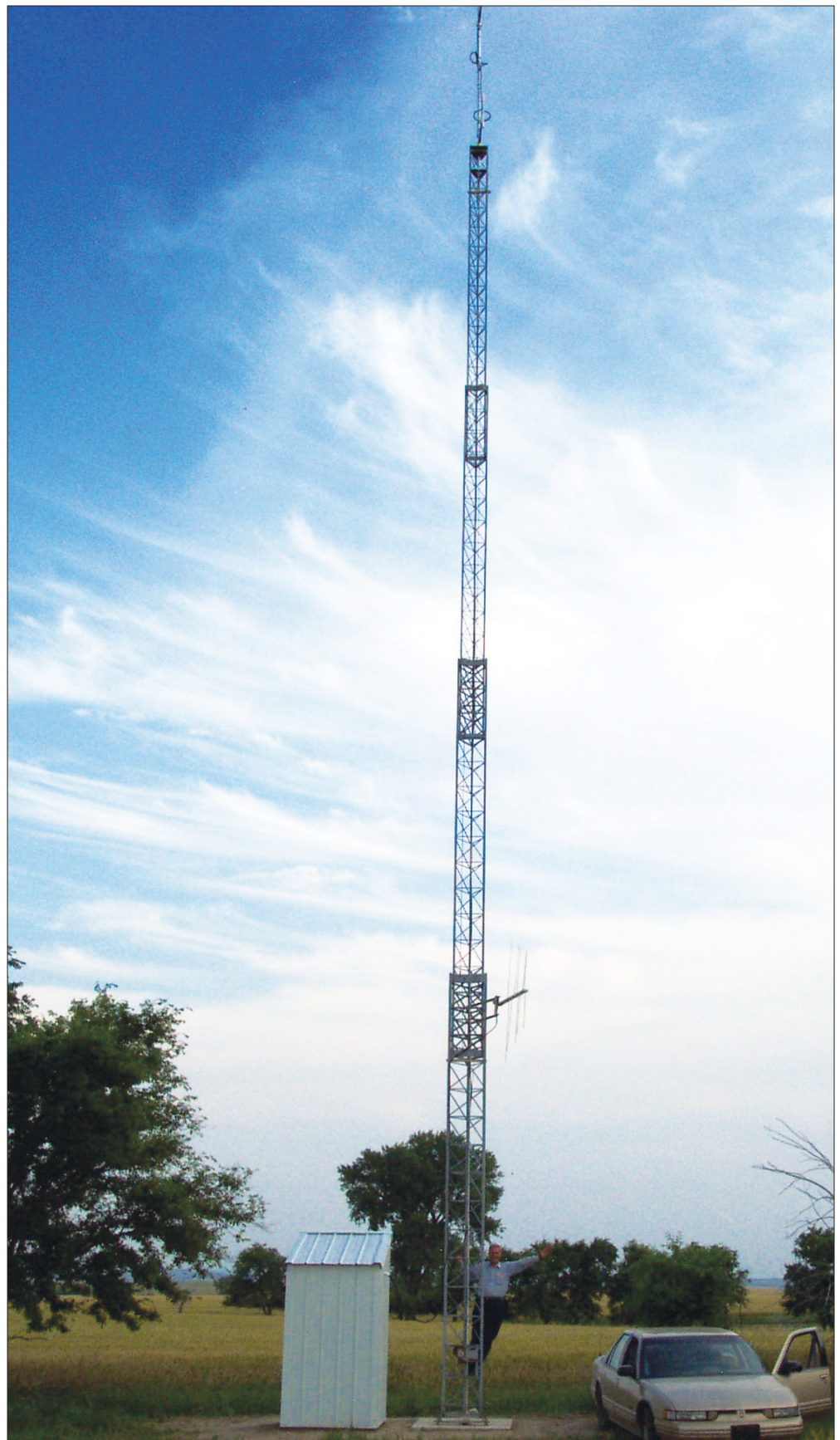
Ron Myers of Radio 74 at the completed KJIT translator tower
