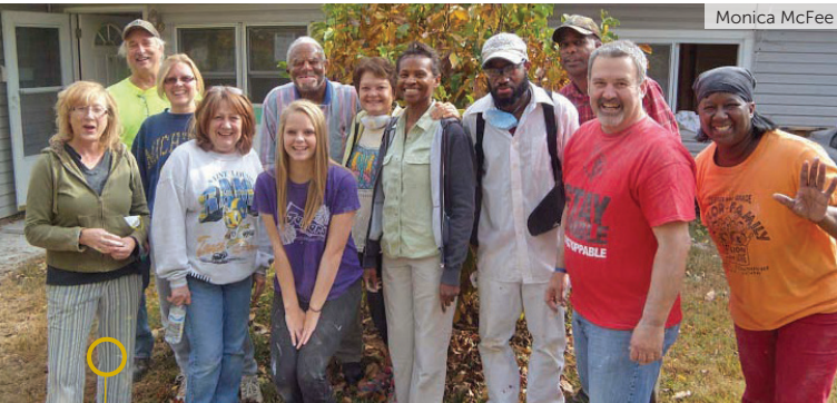
A team of volunteers from St. Louis repainted the interior of a needy family's home, making it possible for the rest of the home to be repaired.
