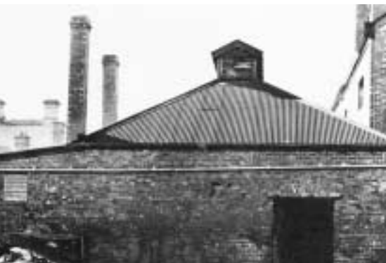
The first factory, Northcote, Vic.
