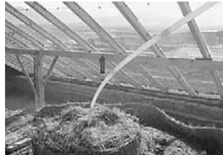
Insulating the biogas plant and placing it in a greenhouse will ensure continued operation even during the coldest winter temperatures.
