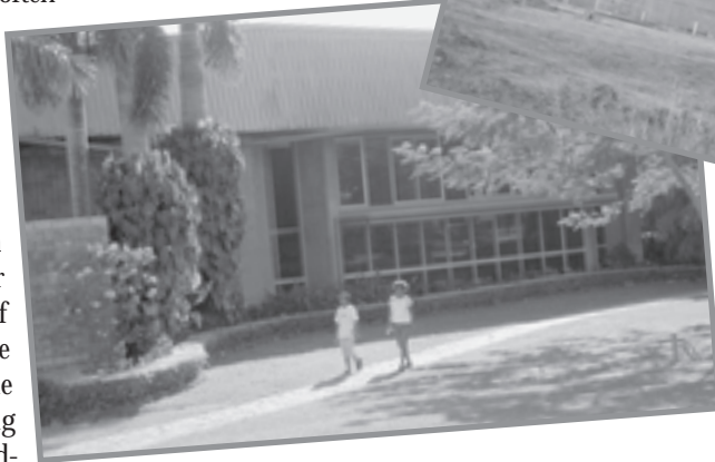
The library at Pacific Adventist University (below) and the new health sciences building taking shape (right).
