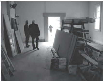
Donated material and equipment clutter the interior of Sunflower House, Wagga Wagga, NSW, which is being refurbished, in part, with funds donated by ADRA—Australia.
