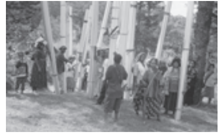
Villagers carry roofing iron for the Algui church, Western Highlands Mission, PNGUM.
