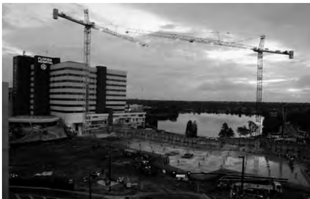
The new foundation at Florida Hospital.
