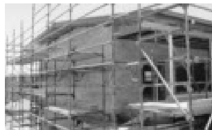
One of the new classrooms at GCCC during its construction.
