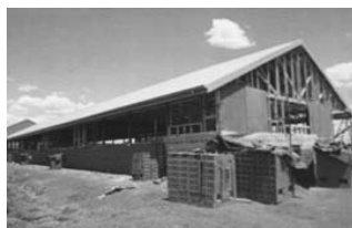
Building work at Border Christian College.
