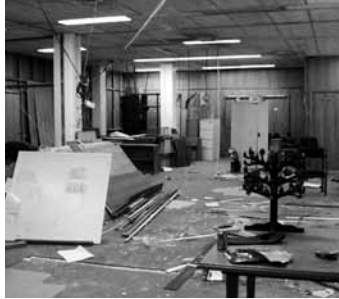
Renovation work underway at Pacific Adventist University's library.
