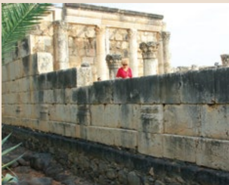
The white fourth century BC Capernaum synagogue is believed to be built on the black basalt foundations of a first century synagogue, which the apostle Luke seems to indicate was built by the centurion whose servant Christ healed.
