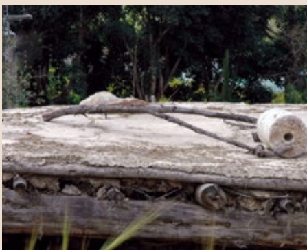
Roofs in the first century AD were often made of layers of plaster and mud laid down over reed mats and placed over branches and logs. Stone rollers compacted the mud. It was through such a roof that the paralytic man was lowered.
