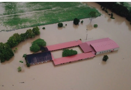
Murwillumbah Adventist Church completely surrounded by flood waters.
