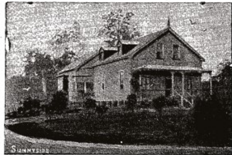
The Home of "Sunnyside."
