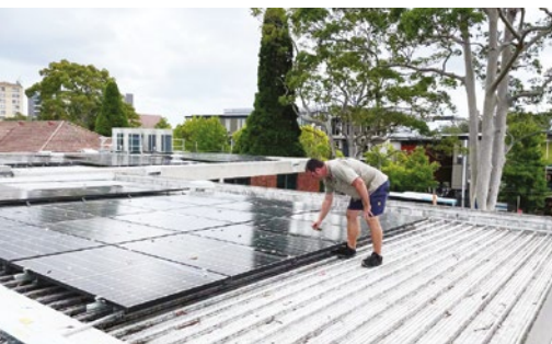
Maintenance supervisor Adrian Wright inspecting the solar panels on the roof of the SPD office.
