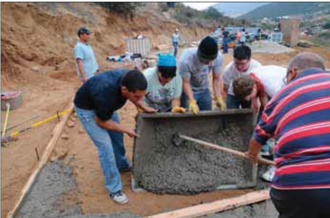
Students from La Sierra Academy pour cement into the foundation form.
