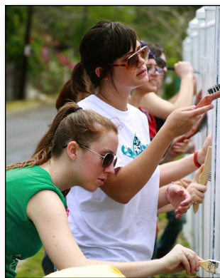
Newbury Park Academy students went on a mission trip to Vieques, Puerto Rico, in March 2011. They painted fences and prepared the foundation for the fellowship hall.
