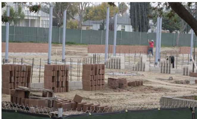
The foundation takes shape during the construction phase.
