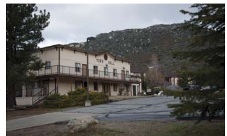
When the Town Hall was completed in 1970, it offered the first hotel-style accommodations at Pine Springs Ranch.
