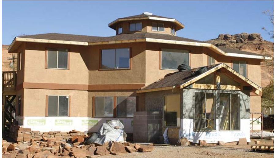
The new health center is currently under construction.
