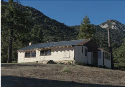
When the PSR property was purchased in 1961, this ranchhouse and a wooden barn (where the pool is now) were the only buildings on site. In 1961, the ranchhouse served as kitchen, dining hall, medical clinic, housing for women's staff and camp store.
