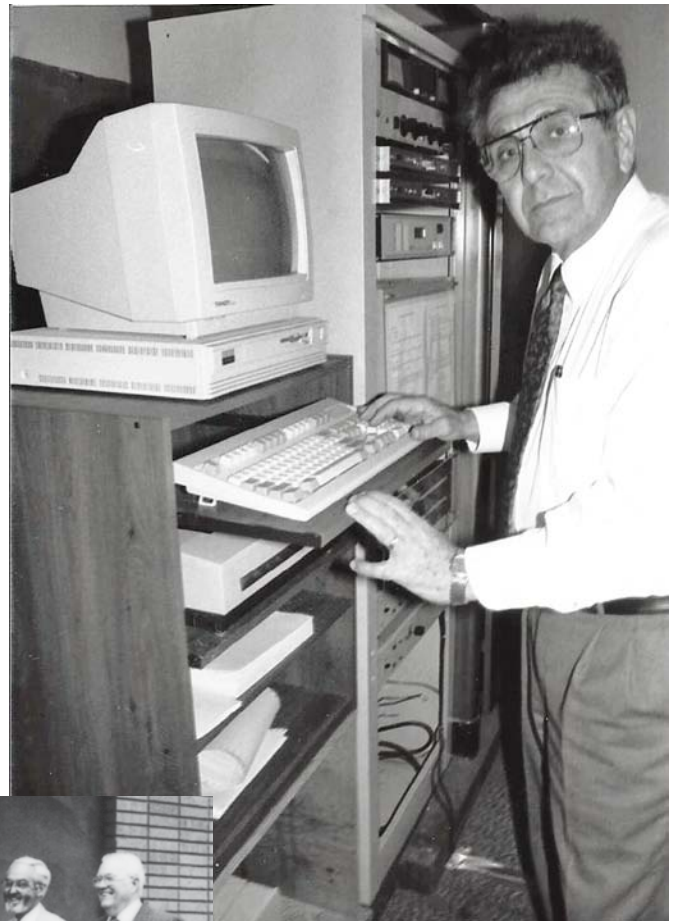
Gaylord Boyer installs equipment at the KADV radio station in the early 1980s. Located on the campus of Central Valley Christian Academy (formerly Modesto Adventist Academy) in Ceres, Calif., the new radio ministry included curriculum and on-air broadcasting experience for the academy students.
