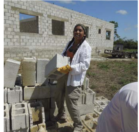
Elyana Martinez hauls cinder blocks at the new orphanage building site.
