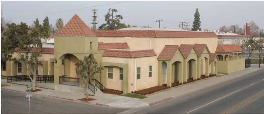
The Fresno Hispanic church on the corner of Olive Avenue and First Street.
