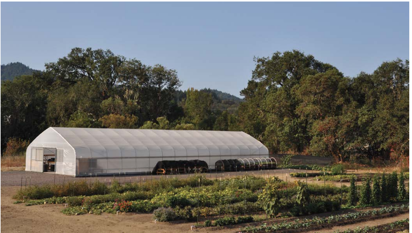
Commonwealth Garden, the 5-acre organic garden project supported by the Howard Foundation to grow produce for the Frank R. Howard Memorial Hospital/ Adventist Health, completed construction of the 30x96 ft. greenhouse in November of 2011. All vegetable crops were started from seed in the greenhouse March 2012, which made it possible for the Garden to provide hundreds of pounds of produce to HMM/AH starting this July. Winter crops are now providing the Hospital kitchen with lettuce, greens, cabbage, broccoli, cauliflower, kohlrabi, and snow peas, along with produce picked and stored from the summer's bountiful harvest.
