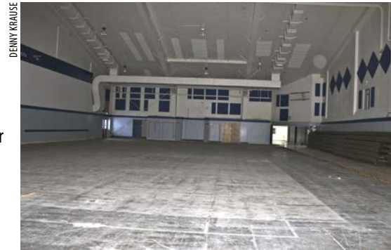
The seller took the wood from the gym floor with them as part of the sale, which left a less-than-ideal play surface.
