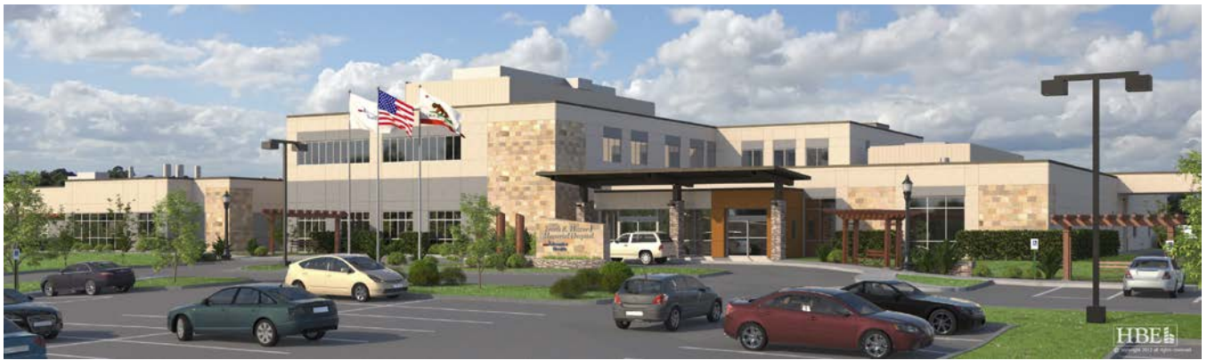
The new Howard Memorial Hospital in Willits, Calif., is scheduled to open in 2015.
