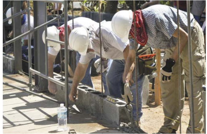
Workers wear the on-site “uniform”: hard hats and neck kerchiefs.
