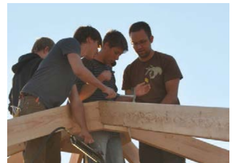
Volunteers relied on teamwork to make the project come together.
