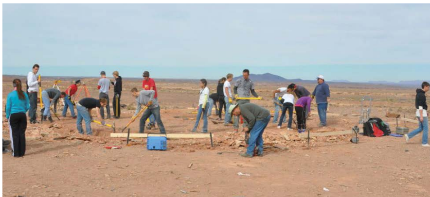
Students clear the ground before pouring the foundation.
