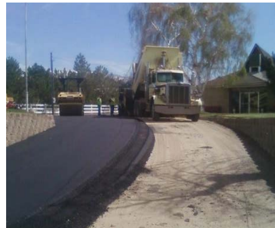
Members and contractors lay the asphalt for the new parking lot.
