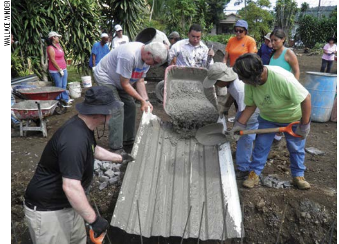
Kerby Oberg, Steve McClain and Norah Castro guide concrete into the channel.
