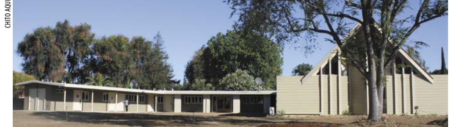
The Livermore church added classrooms (left) and remodeled the fellowship hall (center).
