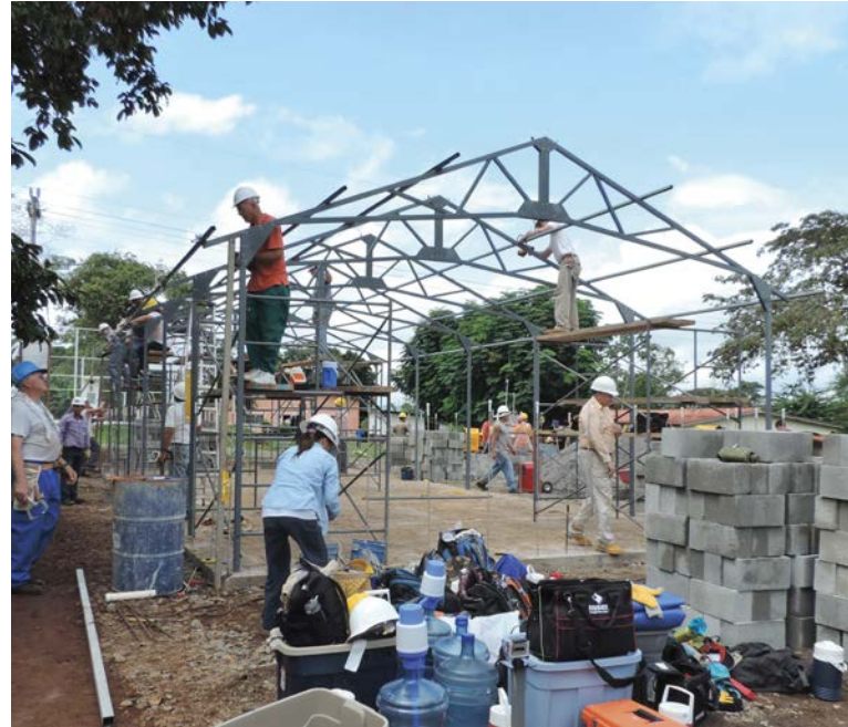
Mission trip attendees work on one of the two building sites.
