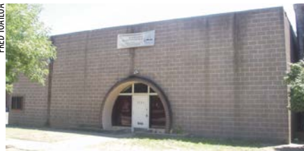
Before: the Sacramento Samoan church met in a warehouse.
