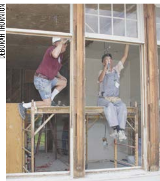
Volunteers remodel a classroom at Sacramento Adventist Academy.
