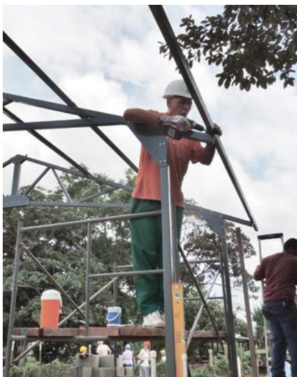
A member of the Corona mission team helps construct a One-Day Church building.
