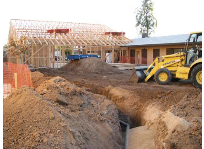
The project tripled the size of the fellowship hall.
