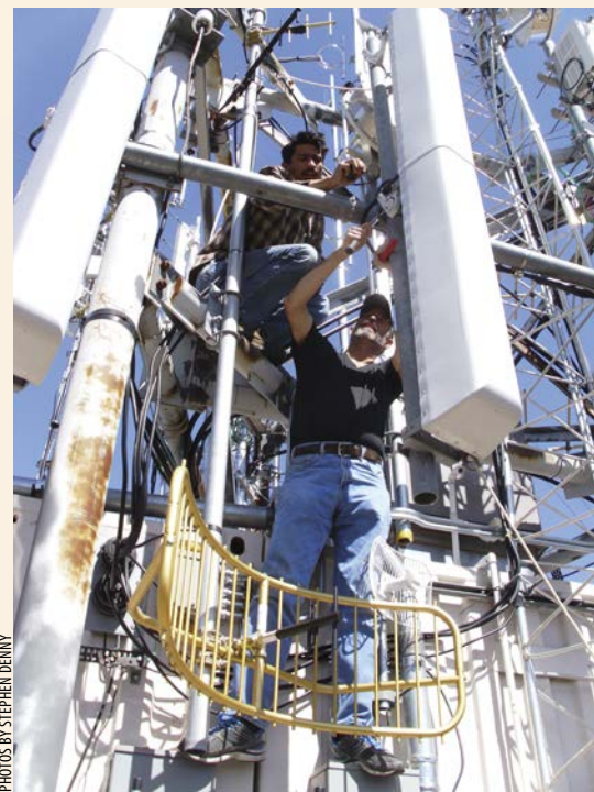
GNTV crew members Moses Tyler and Leland Preston rigging TV broadcast antenna on the Payson tower site.
